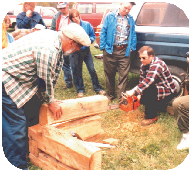
Bill Koski showing how to right the corners of replacement logs
