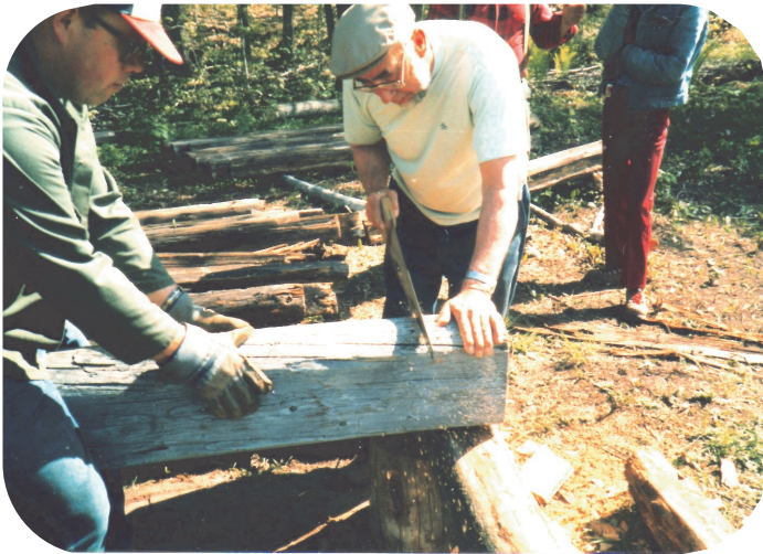
Bill Koski showing how to right the corners of replacement logs
